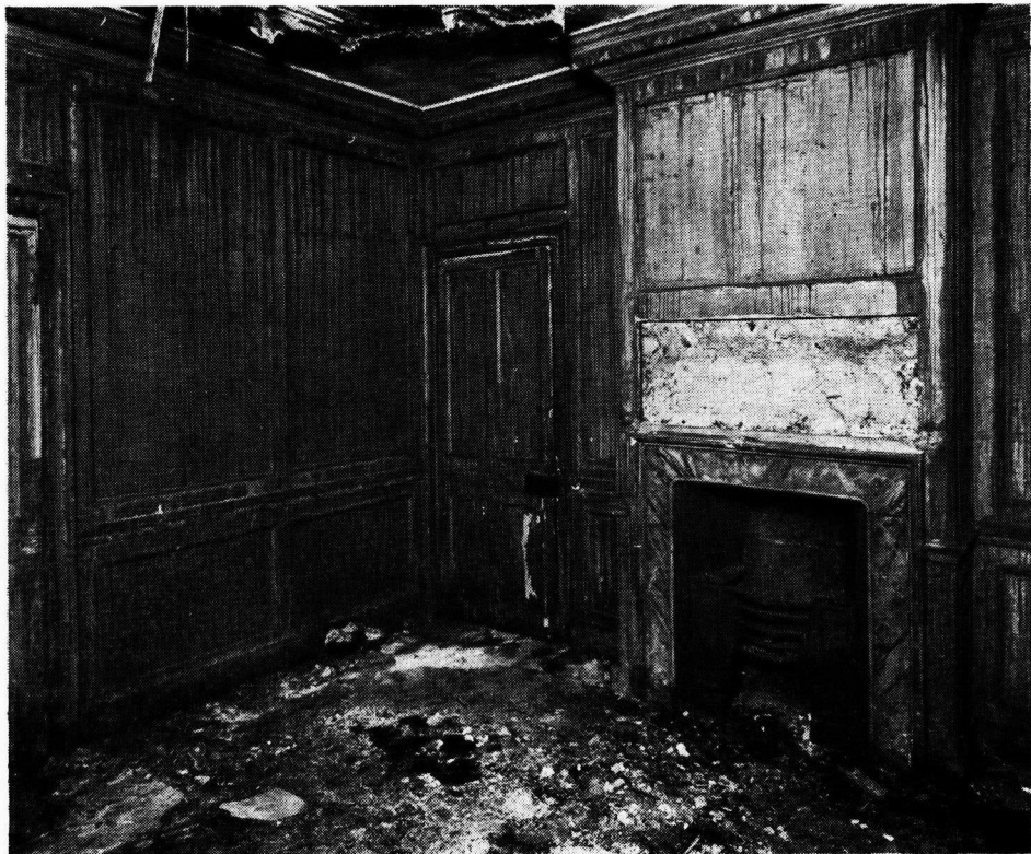
NO. 38 NORTH END CRESCENT, FULHAM. First floor front room (south-east)
