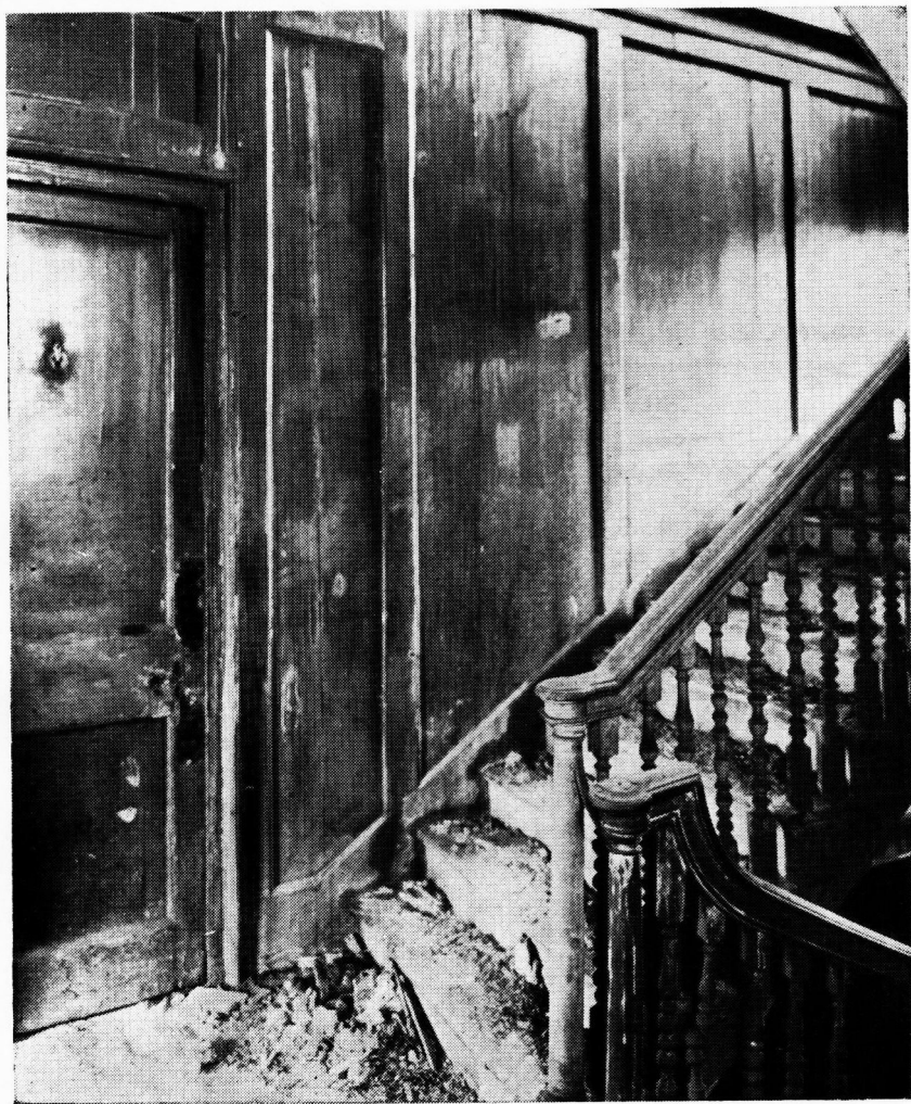
NO. 38 NORTH END CRESCENT, FULHAM Staircase at first floor
