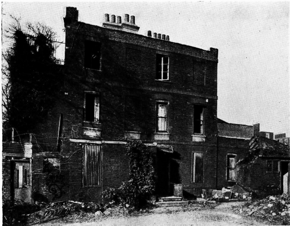
NO. 38 NORTH END CRESCENT, FULHAM South-east flank
